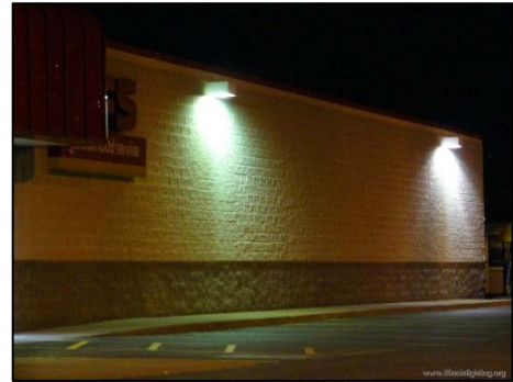
Figure 6.2. Building lighting directed downward
