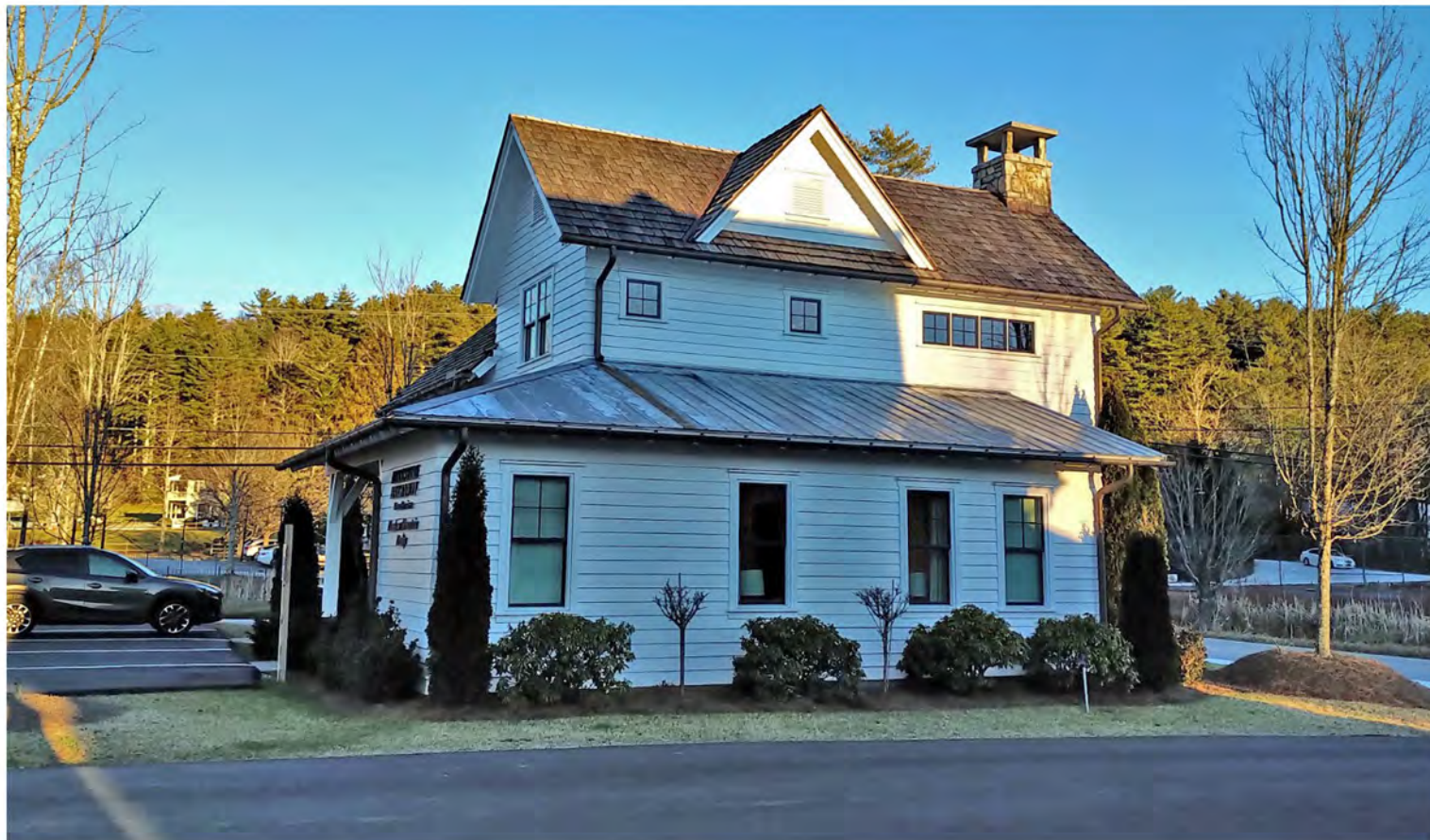
A newly constructed two-storied commercial building in Cashiers featuring vernacular wood siding.
