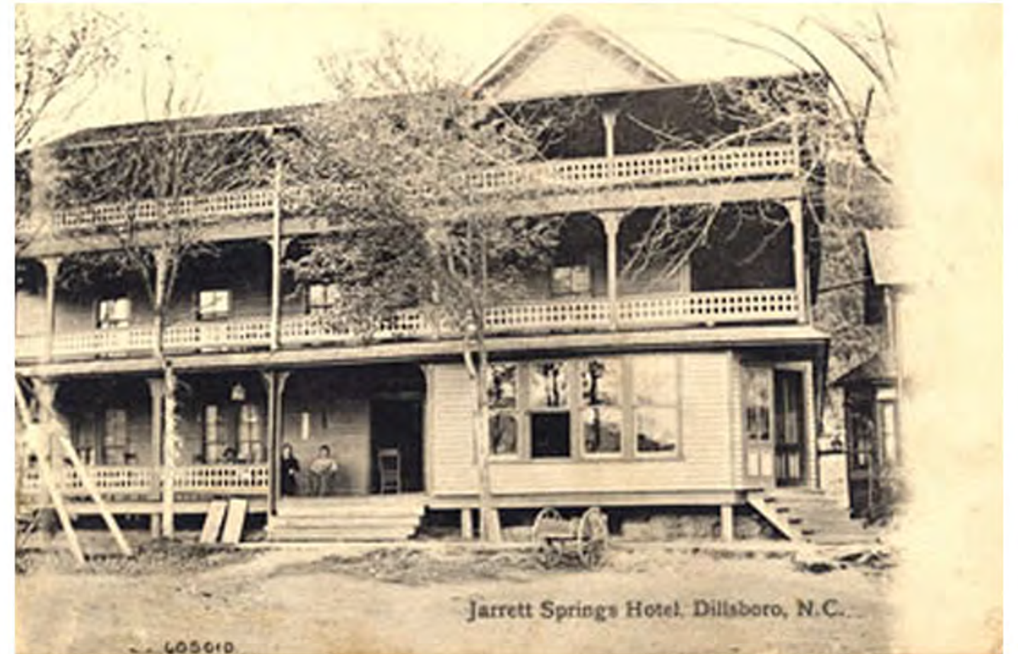
The Jarrett Springs Hotel in Dillsboro, North Carolina, c. 1884.
