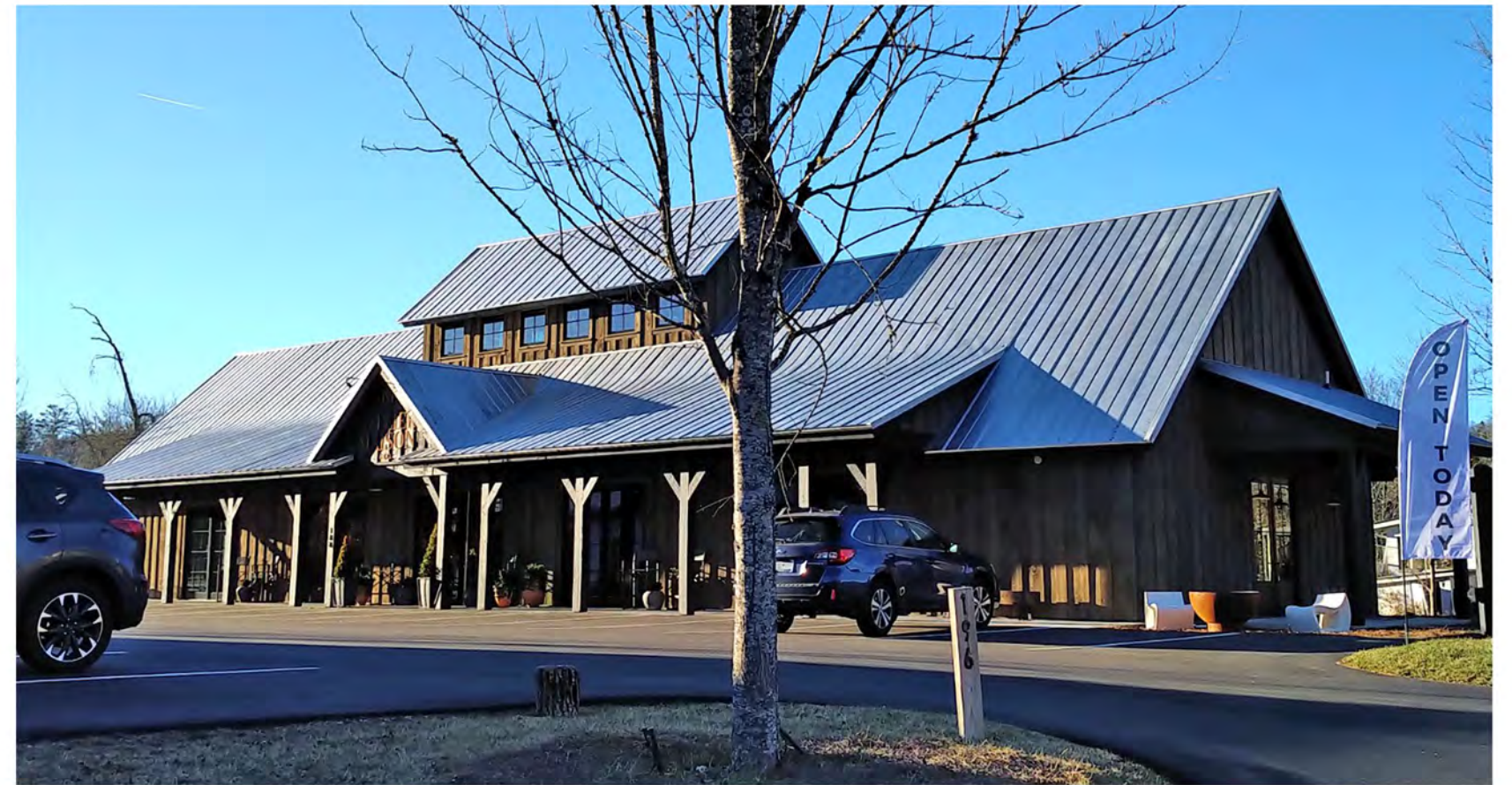
Commercial space in Cashiers with simple roof forms and timber support beams.
