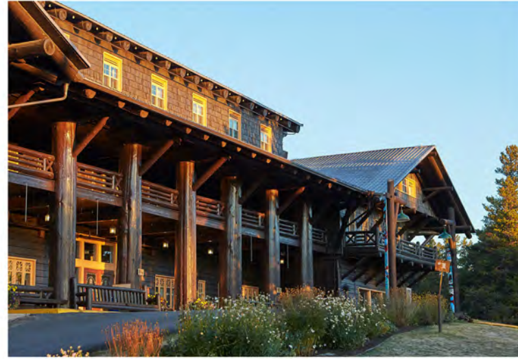
A generous portico welcomes visitors to this historic park lodge.
