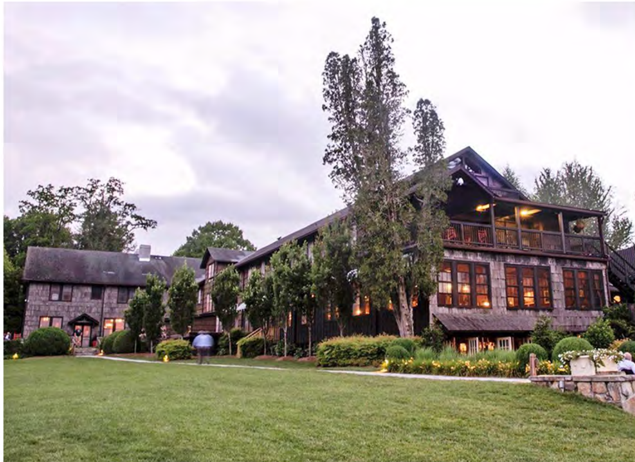
Chestnut siding is a signature material that defines the majority of the facade at the High Hampton Inn.
