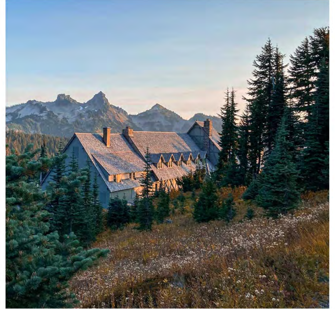
Shed roof forms and gabled dormers are part of a distinct mountain vernacular.
