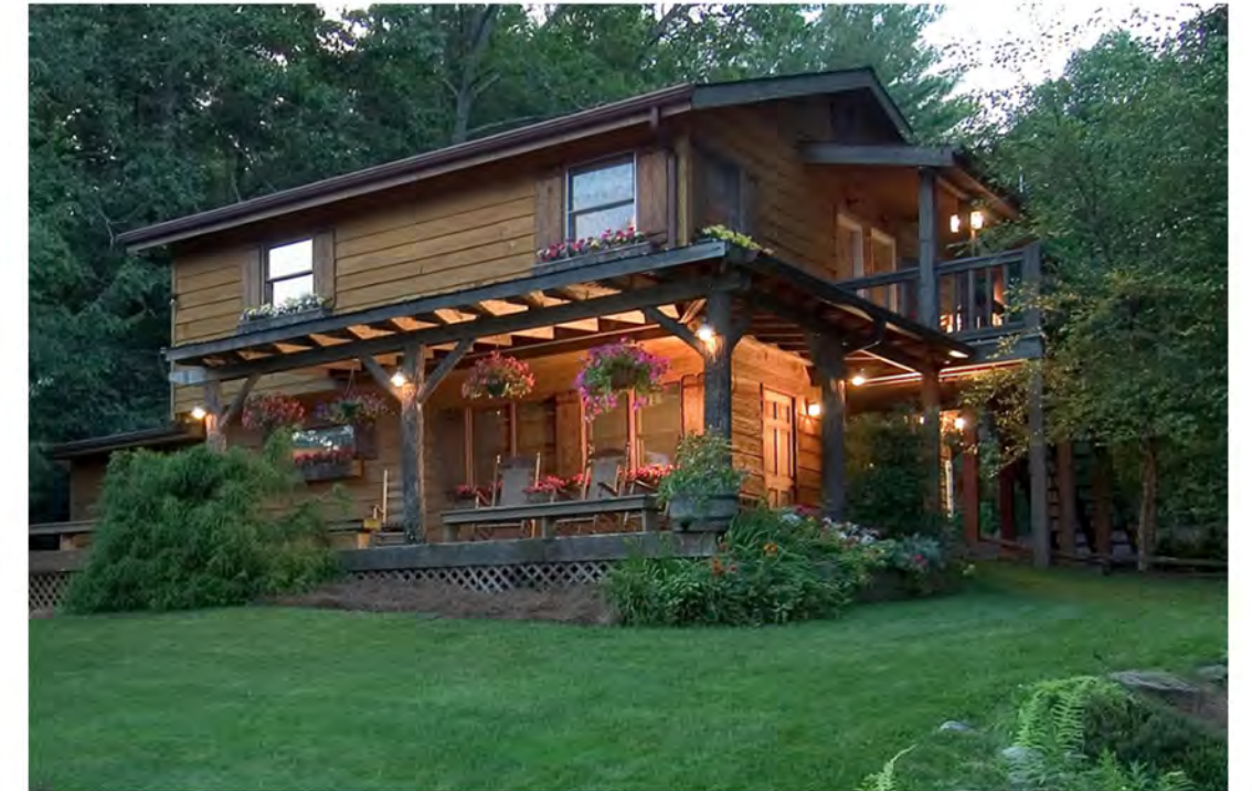
The Laurelwood Mountain Inn on Highway 107.
