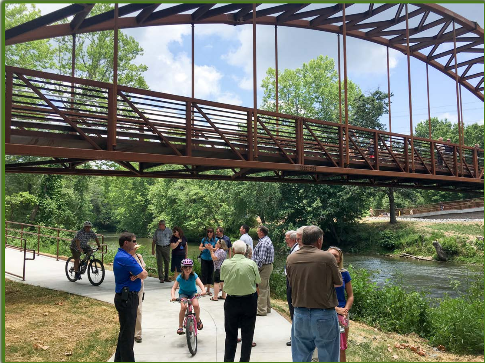
Pedestrian Bridge on the Greenway in Cullowhee Photo Courtesy of Nick Breedlove
