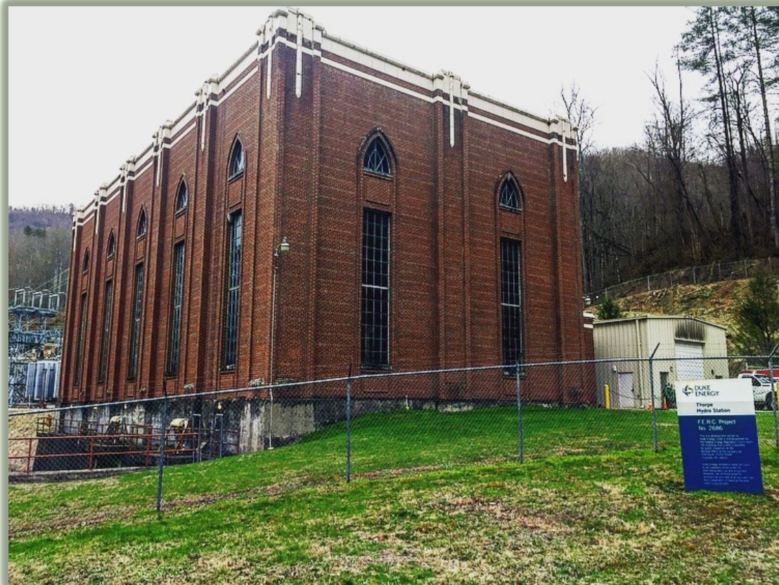
Duke Energy Hydro Station, Photo courtesy of Caroline Edmonds
